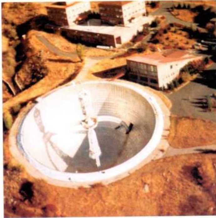
a - General view from helicopter
